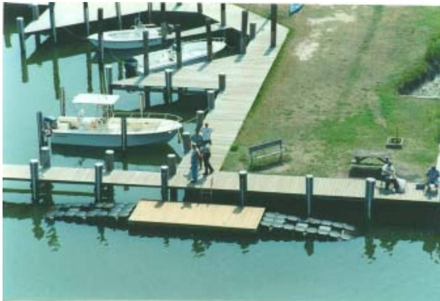
Photo 5E: At Janes Island’s busy marina, the floating launch provides access to paddlers at a safe distance from heavy motor boating traffic
