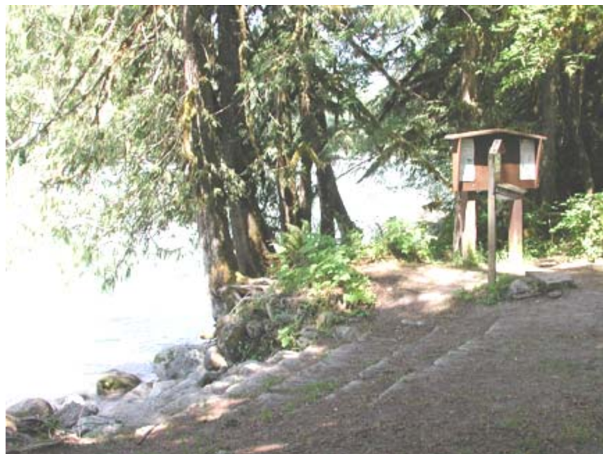
Photos 9F, 9G: Rock staircase provides river access with a “natural” appearance
