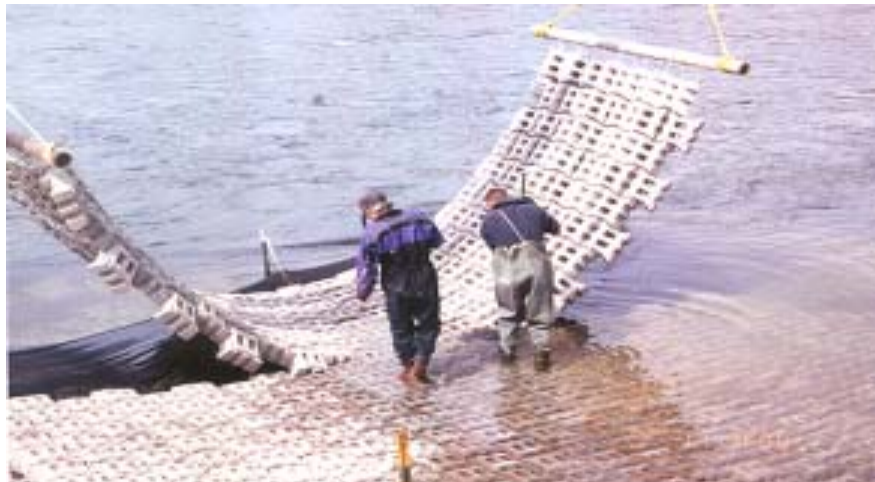
Photo 8K: Crane is used to place and interlock mats
