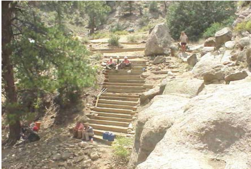
Photo 9D: Rectangular timber stairs with varying treads provide access to steep shoreline while helping to mitigate erosion
